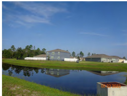
Pond 11: Pond in good condition.
